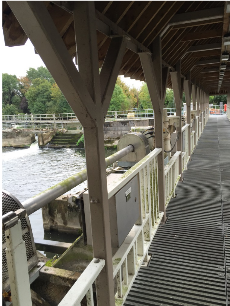
Fig 9: Existing private footbridge structure crossing the weir.
